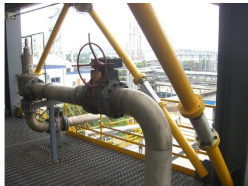
Fig. 6. Frame structure damper arrangement
